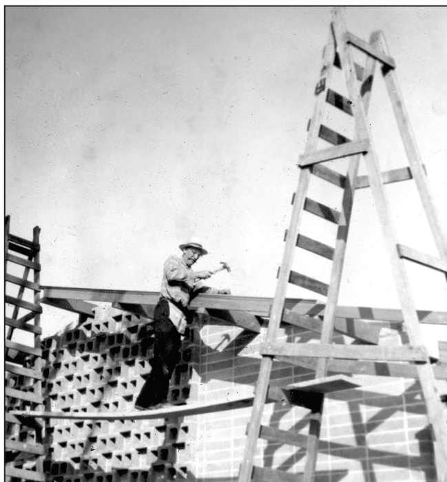
Dad working on Ballarat Chapel
